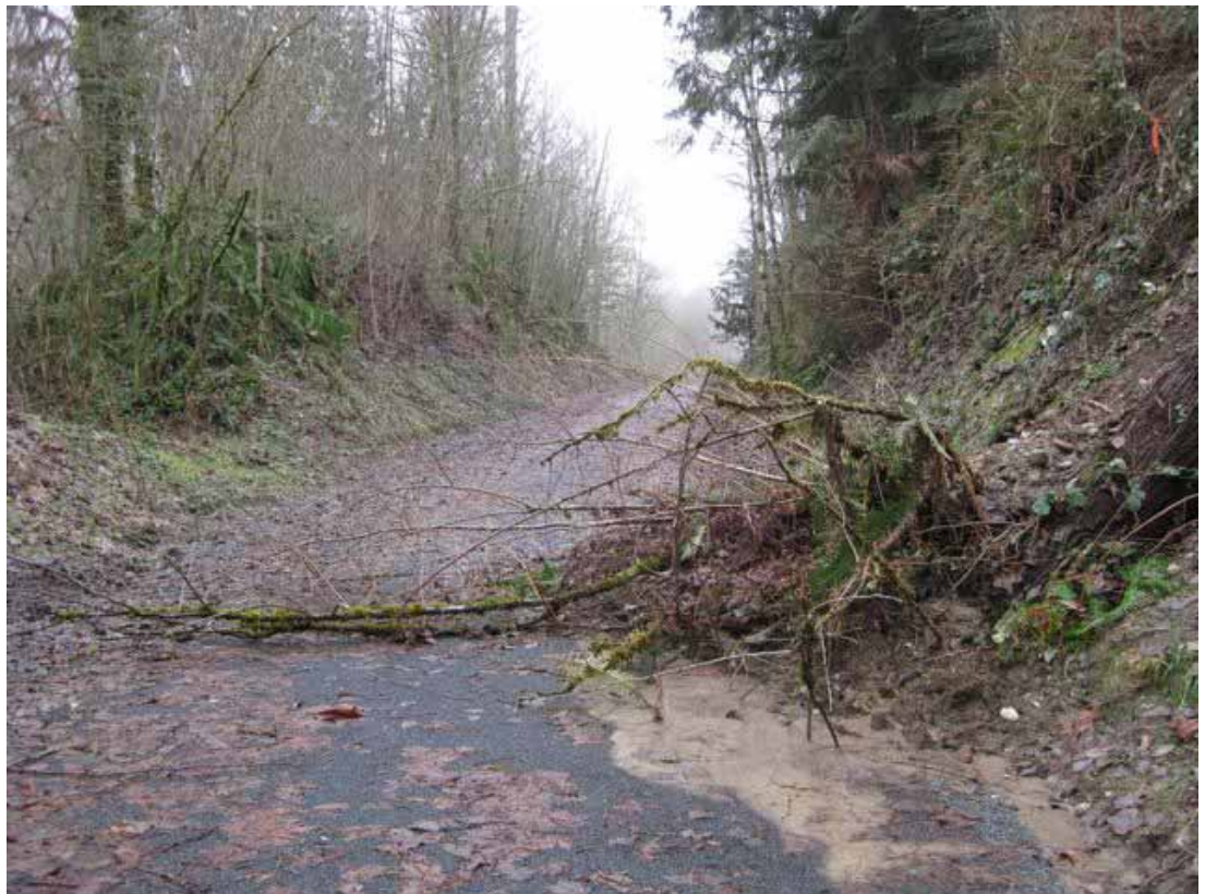
Right: "There were a few minor earth slides covering the new pavement."
